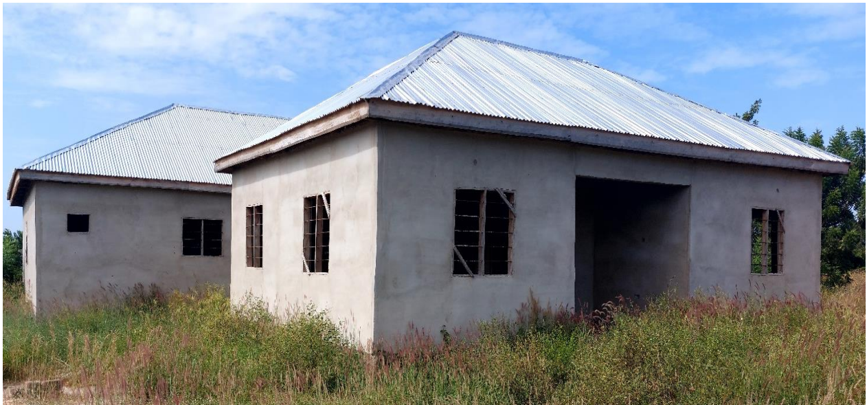
Photo 19: Construction of CHPS compound and 1No. semidetached staff bungalow at Gumo
