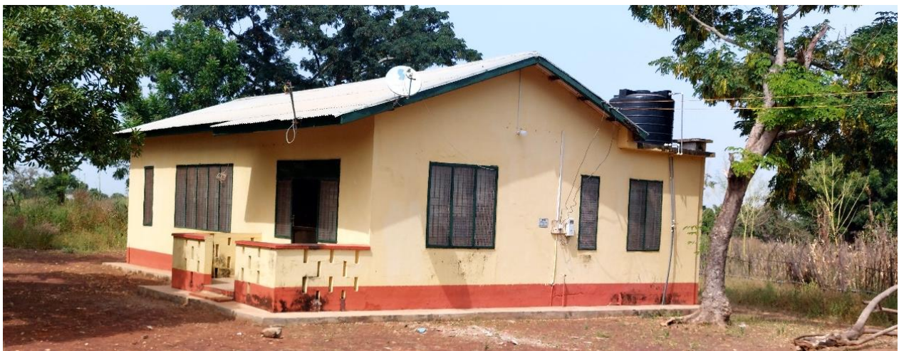
Photos 6-8: Rehabilitation of 3no. staff quarters at Savelugu
