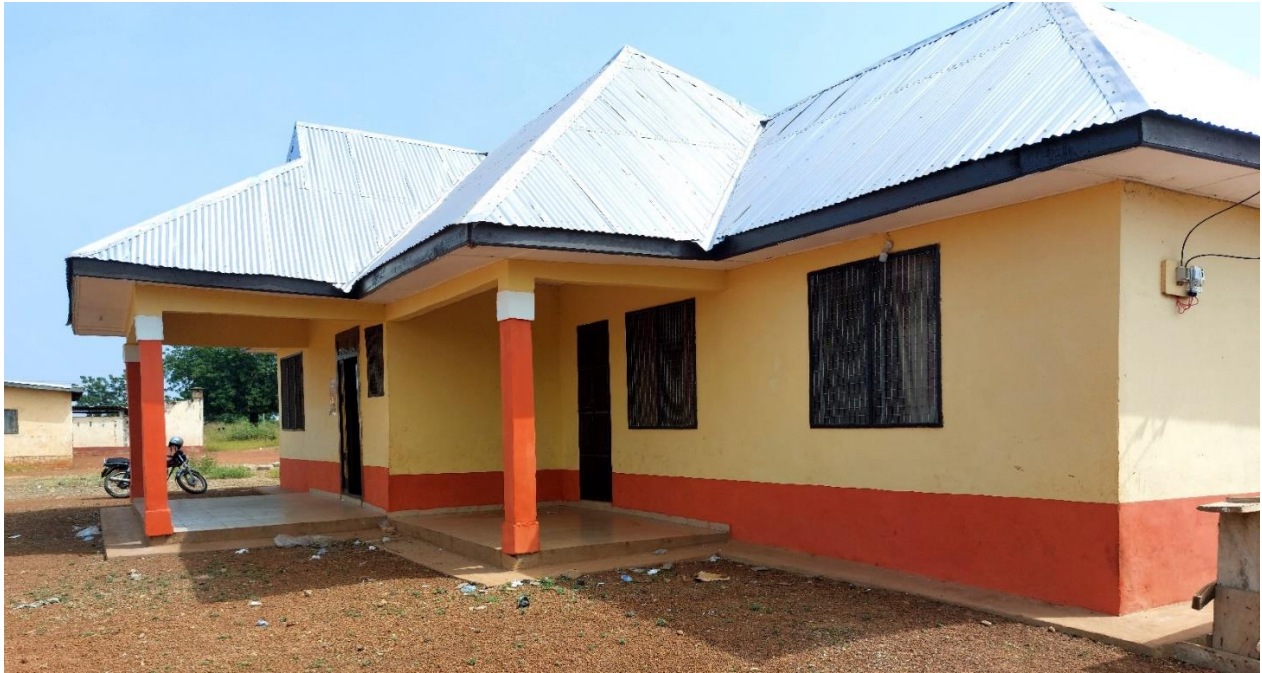
Photo 18: Construction of 1No. CHPS compound at Kanshegu
