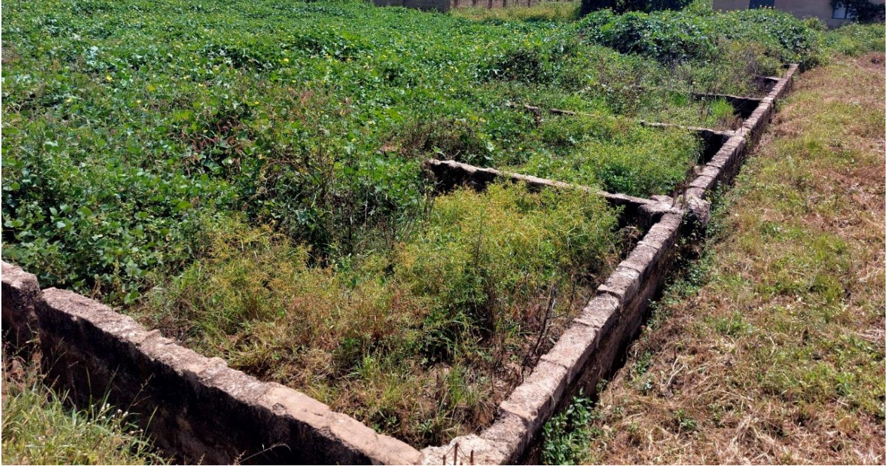
Photo 3: Construction of 6-unit classroom block at Nuri-Imaam primary school
