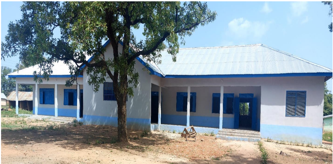
Photo 15: Construction of 1 No. 3 unit classroom block at Nabori
