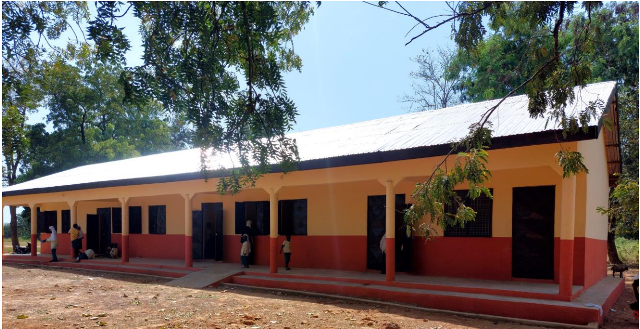
Photo 14: Construction and furnishing of 1No. 3-unit classroom block at Zohe
