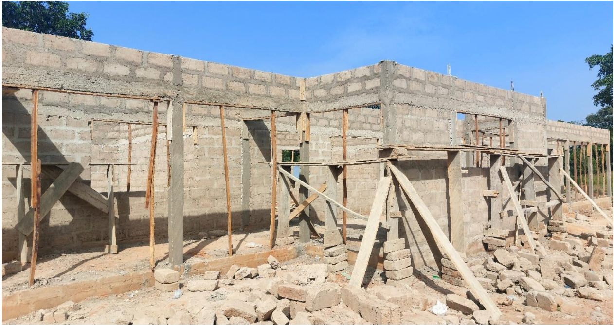
Photo 16: Construction of vocational school at Damongo
