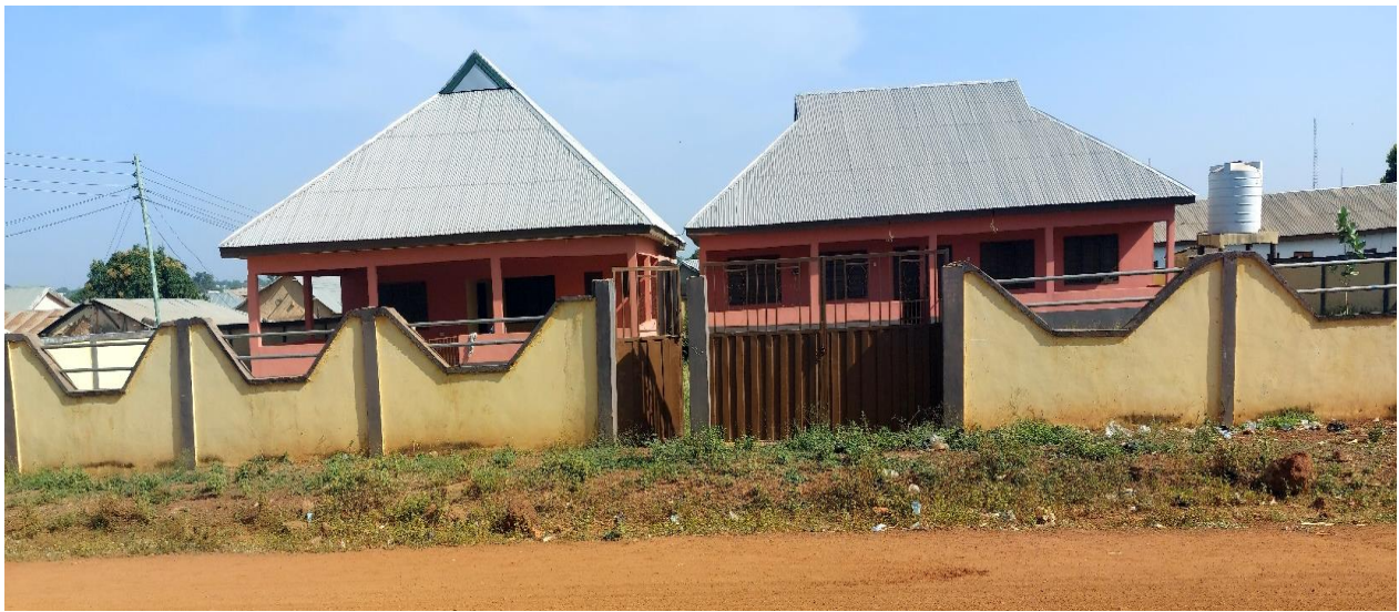
Photo 13: Construction of fence wall, Tiling and furnishing of Wari-Yapala CHPS Compound
