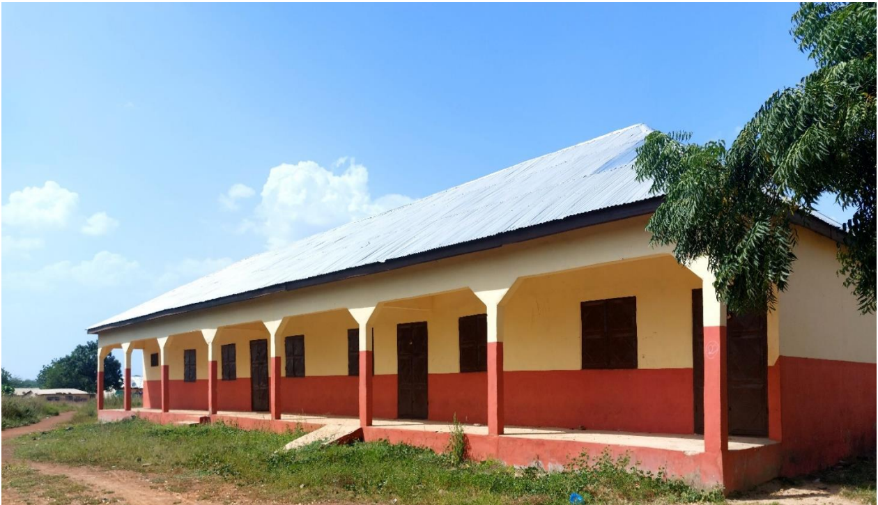
Photo 4: 3-unit classroom and 1-unit office block at Sugashie
