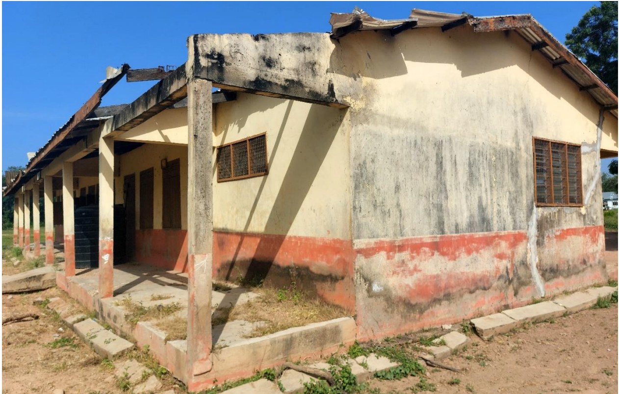
Photo 5: Renovation of 3-unit classroom block at Mempeasem
