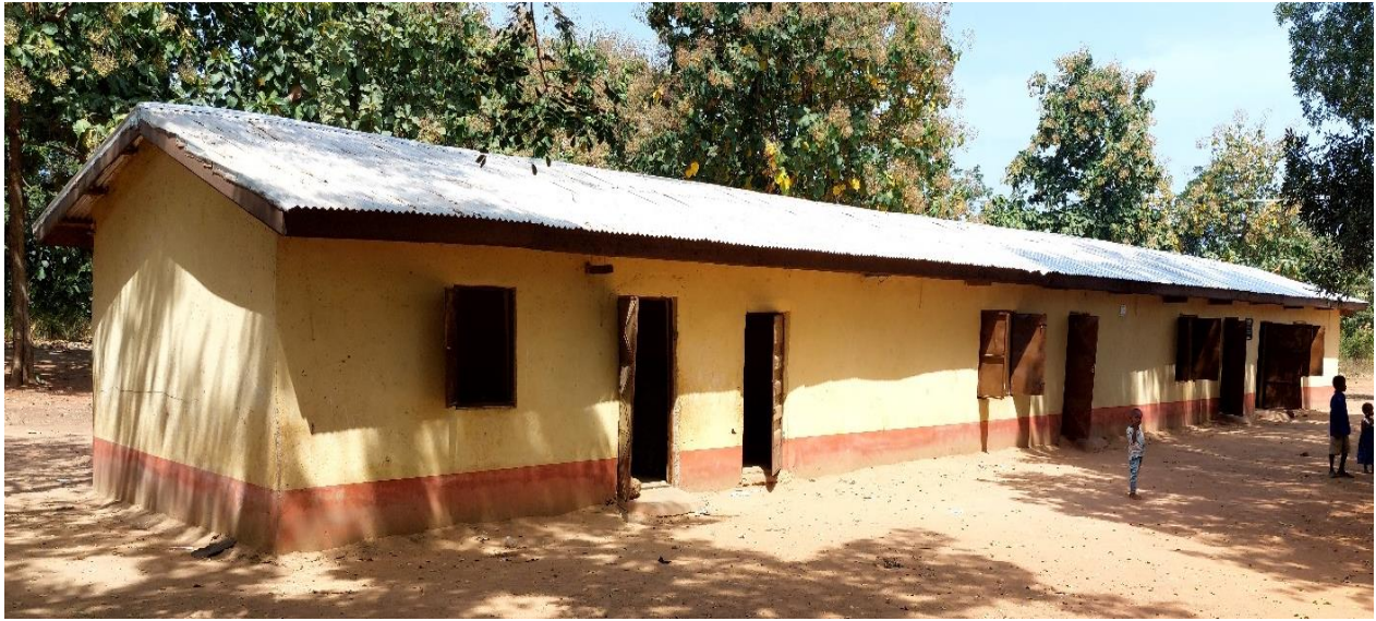
Photo 10: Renovation of a 3unit classroom block at Gbambaya
