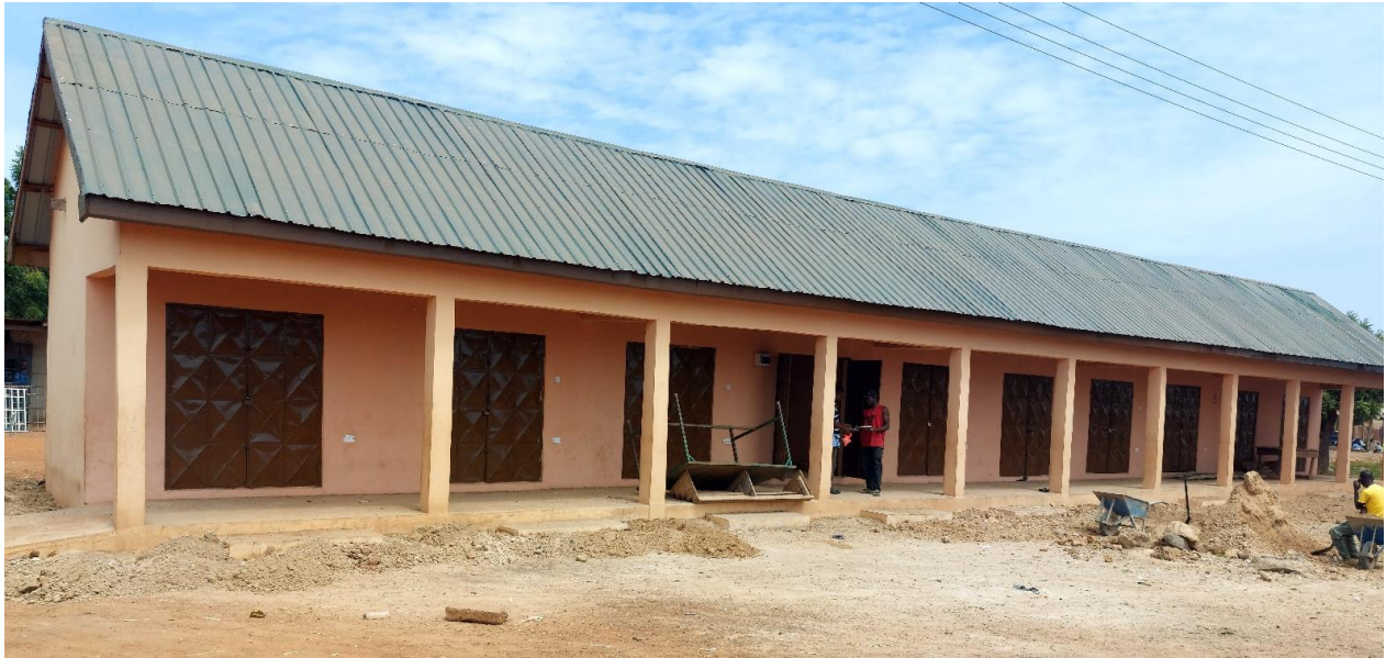
Photo 12: Construction of 10-unit market stalls at Nyankpala
