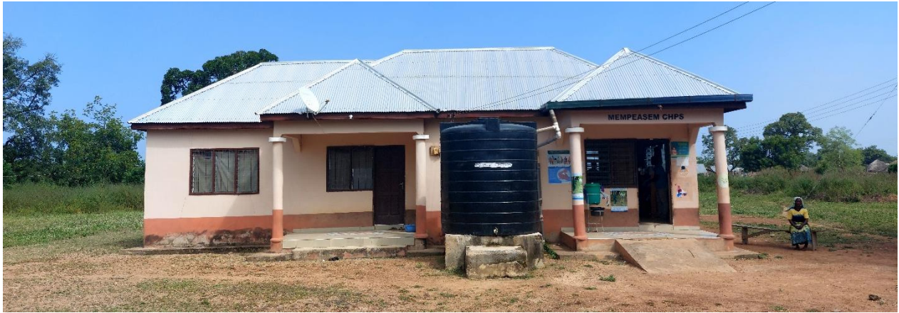
Photo 20: Construction of CHPS compound and 1No. semidetached staff bungalow
